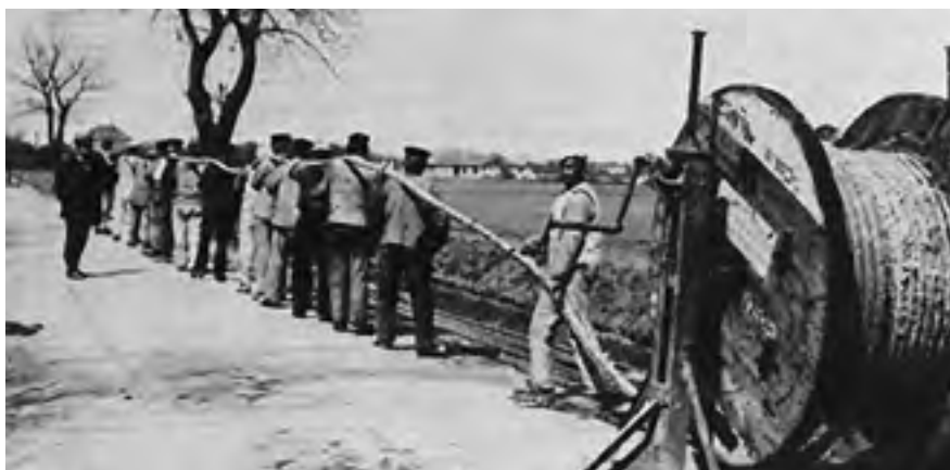
AC cable being laid between Skovshoved and Lyngby.
